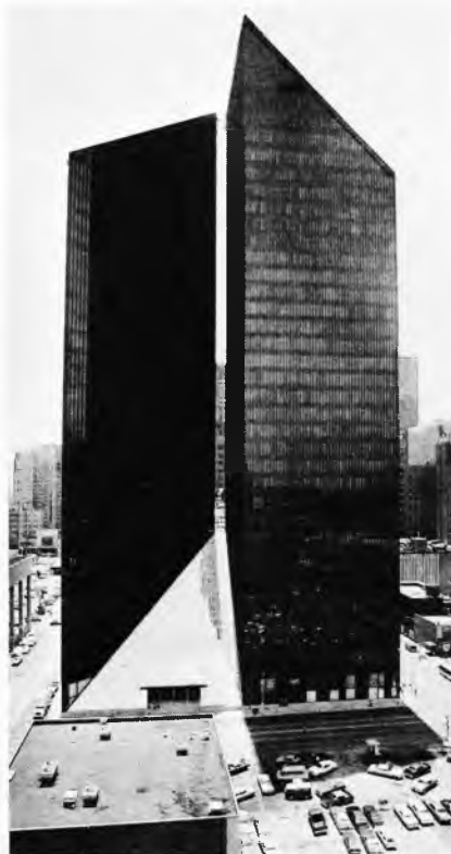
Sl. 45. Tornjevi blizanci Pennzoil Place, Houston; Ph. Johnson i J. Burgee, 1976.
