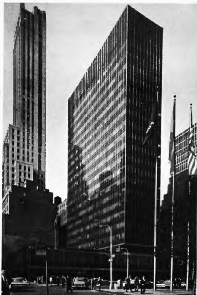
Sl. 38. Lever House, Park Avenue, New York; L. Skidmore, N. Owings i J. Merrill, 1951–1952.
