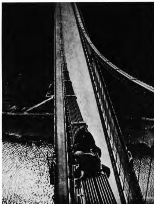
Sl. 15. Pogled na lance mosta Clifton Bridge (sl. 13)
