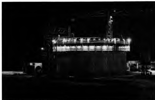
Sl. 16. Bunar strojarnice HE Obrovac s kliznom oplatom
